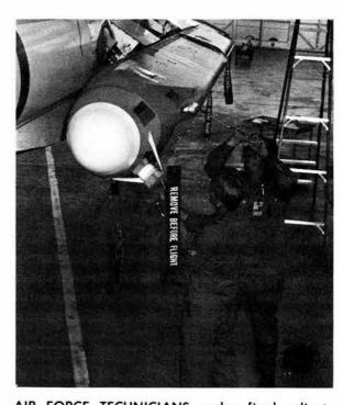
AIR FORCE TECHNICIANS make final adjustments as they mount a Boeing-built Air Launch Cruise Missile under the wing of a B-52 aircraft. Production model ALCMs will carry Sandiadesigned W80 nuclear warheads.
